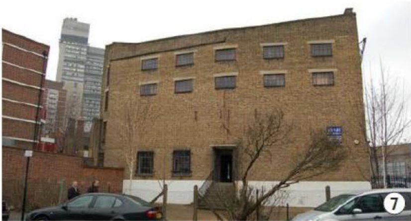
From Hardwidge Street towards the Leather Warehouse
