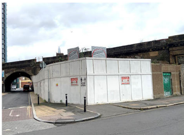
Looking north from the junction of Tiverton Street and Rockingham Street
